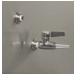
Service Valves/Couplings [Gas, Air, Vac]
