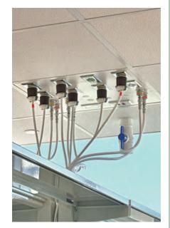
Ceiling Interface Panels [CIPs] are configured to the exact requirements of your lab; with the ability to accommodate future expansions.
